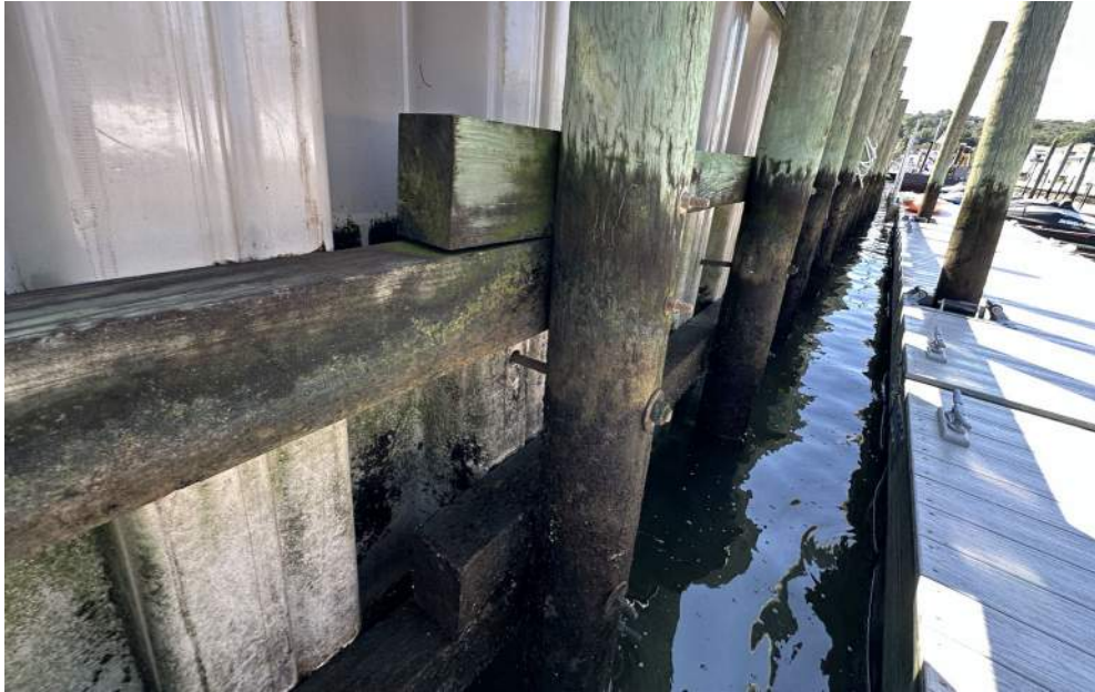
Photo 6: Section A , Easternly Bulkhead Waler Lap Connection, View 2
