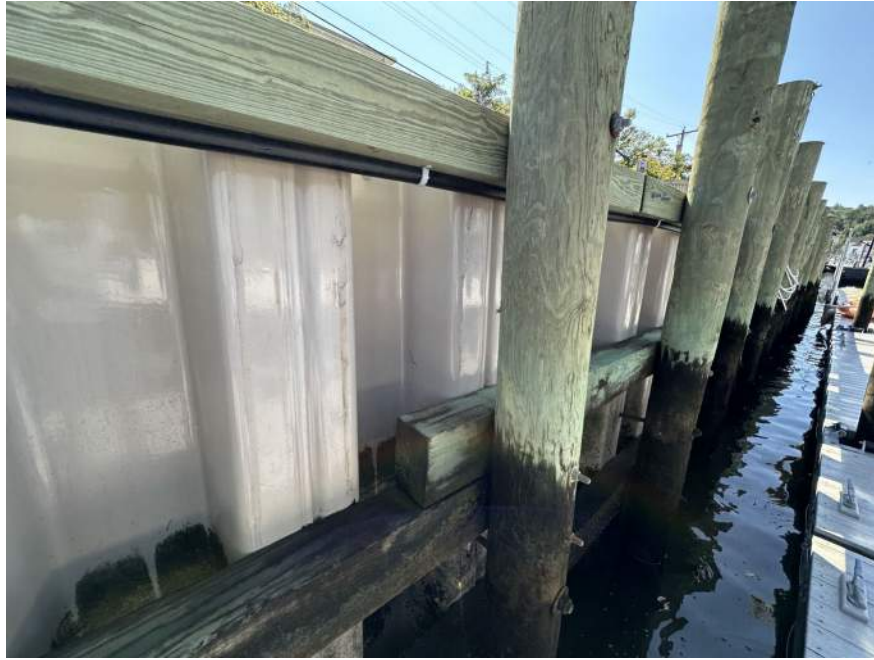
Photo 3: Section A , Easternly Bulkhead Piles, Sheet Piles and Walers Viewed from Floating Dock Infront of Bulkhead
