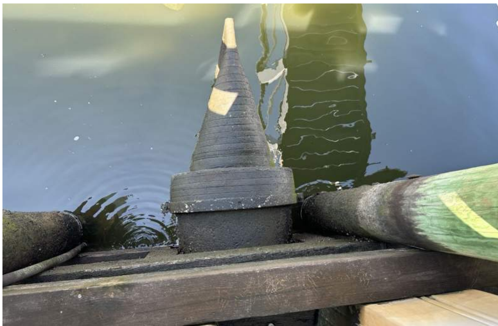
Photo 11: Section A , Eastern Bulkhead, Outfall Pipe with Outfall Backflow Preventer (Tideflex)
