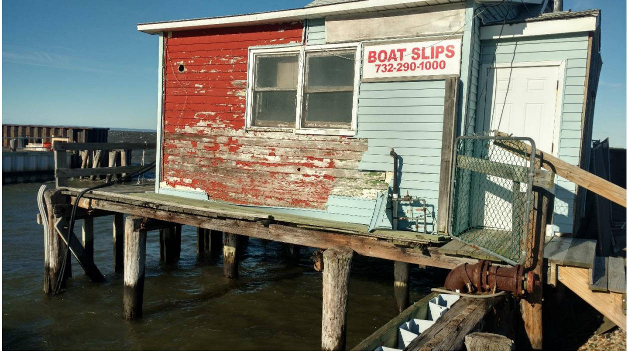
South-facing side of the building, siding damage, walkway damage.
