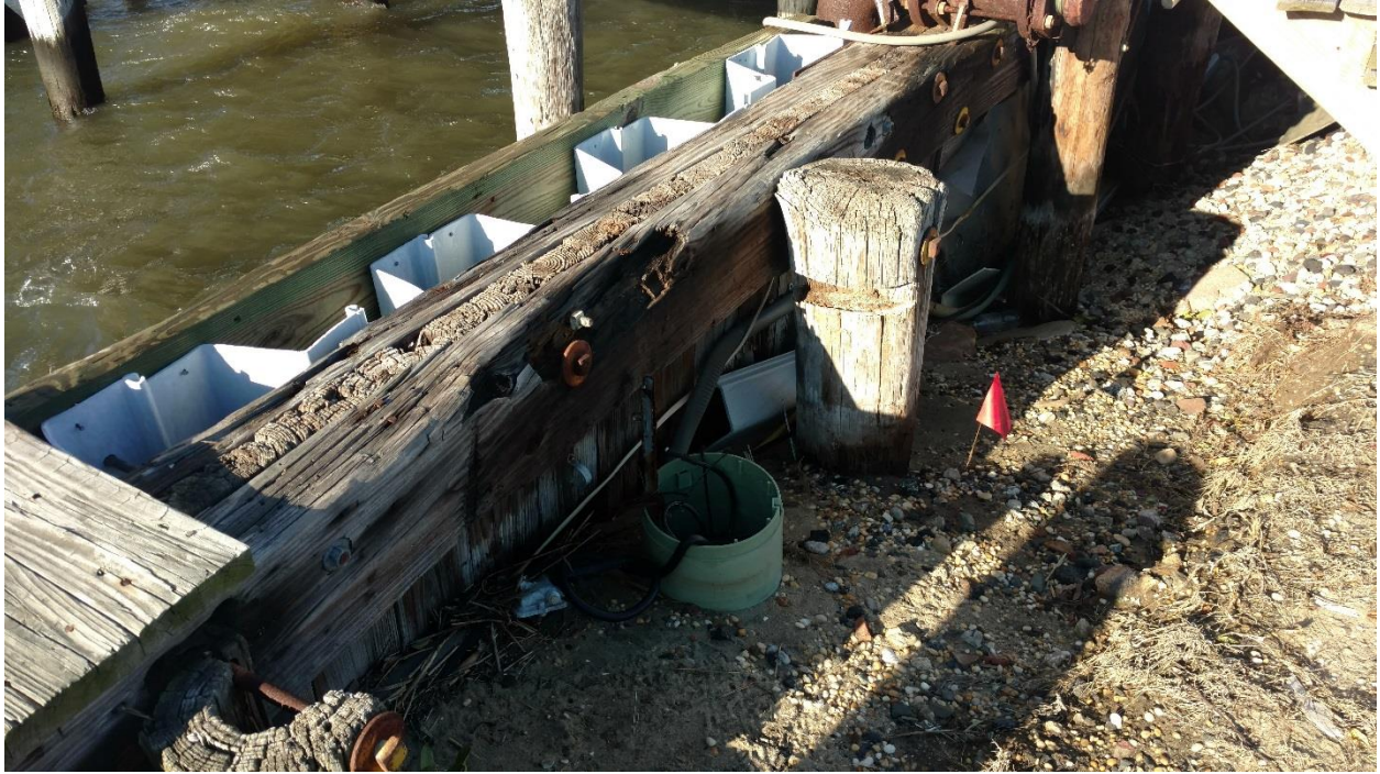
Bulkhead in poor condition, ground subsiding.
