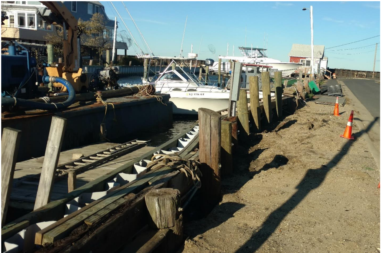
Bulkhead bulging into channel, signs of sand eroding at landward side.
