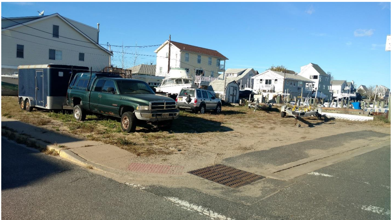
Lot with depressed curb apron, drainage inlet, sand moving off property.
