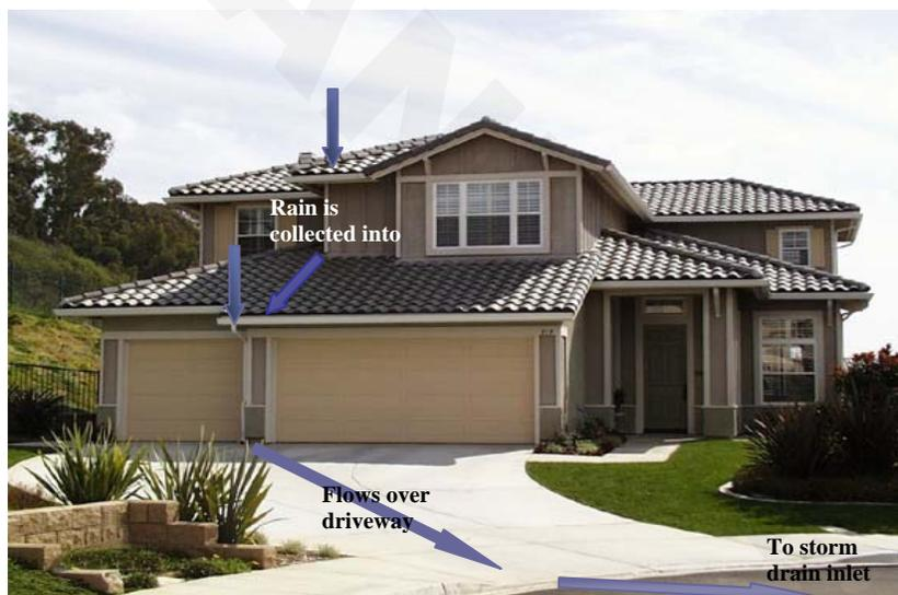
Rainwater is intercepted by roofing and collected into gutters. The water then discharges from the downspout onto a paved driveway and flows to the gutter and storm drain inlets. Alternatively, the collected water is piped underground directly to the storm sewer.
